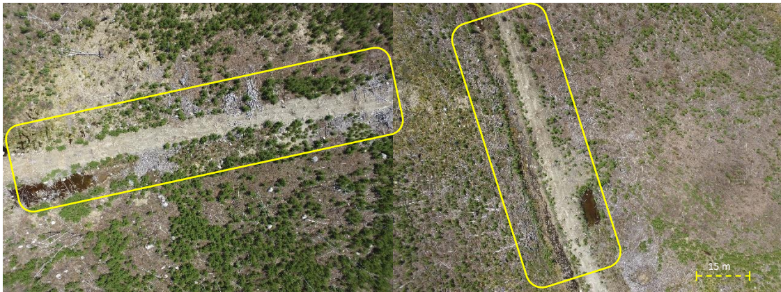
Figure 26. Example of vegetation establishment along road edges. Aerial images were collected in late May 2017 at 120 meters, and the scalloping is visible along the road surface as the lighter and darker swirls that make up the aggregate mounds and troughs.
