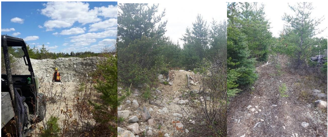
Figure 27. An example of road closure/deactivation (left) and the cut trail subverting it (center and right). The deactivation trench was put in place attempting to prevent access beyond this point, into the central area.
