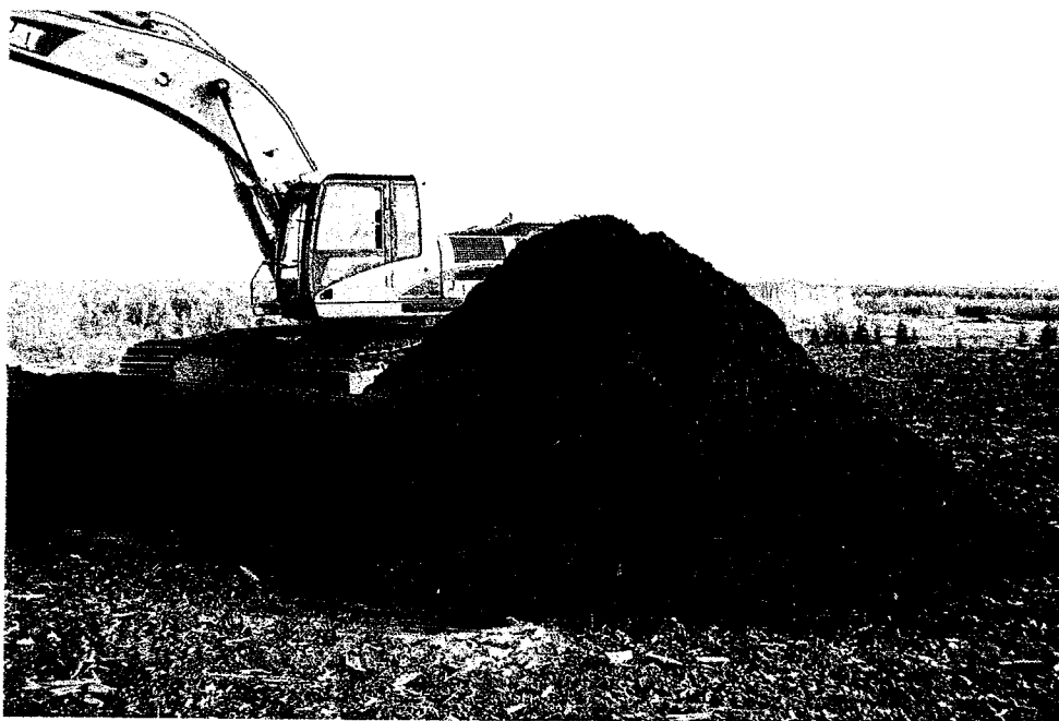
Figure 5.5: View facing north at test pit TP6 material from 4 m below ground surface.
