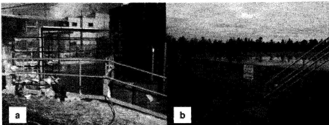
Figure 12 - Effluent collection points for experiments #4 and #5: a – untreated kraft effluent collected from the acid-alkaline sewer. b – secondary treated kraft effluent collected from the #1 kraft secondary clarifier
