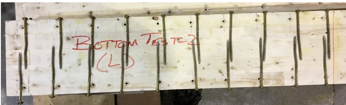
(b) Yielding in bottom screws due to excessive shear stress
