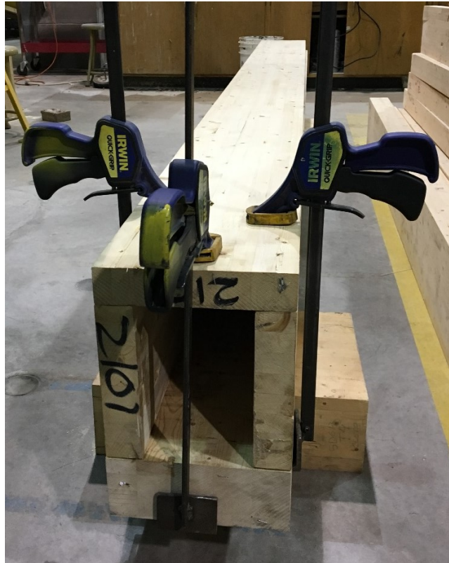
Figure 3.19. Placement of web and top and bottom flange panels
