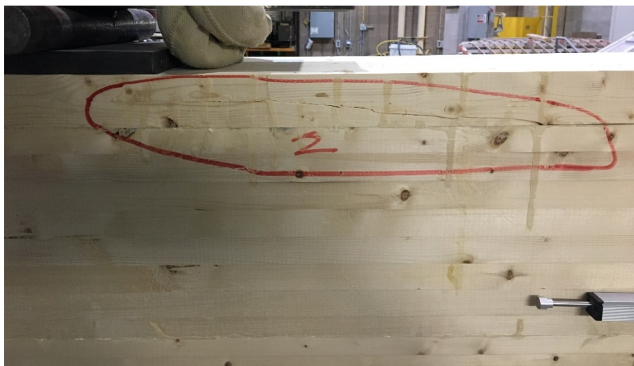
Figure 4.13. Rolling shear failure in the top flange of a general glued beam test assembly
