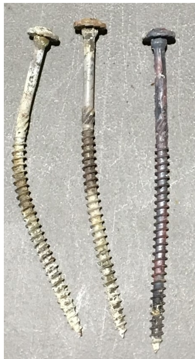
(b) Excessive yielding in bottom screws due to excessive shear stresses and fire exposure
