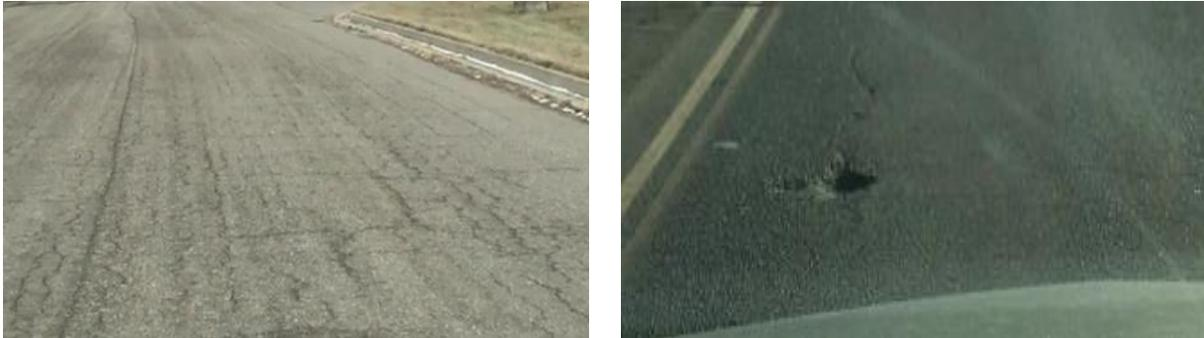
**Figure 6. Road surface texture at different scales. Left: A rough surface with small-scale regularity; Right: An irregular road with a mix of roughness features at different scales**
