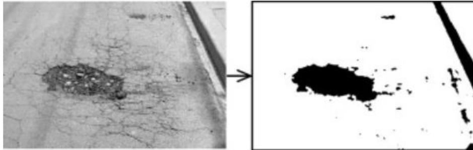
**Figure 14. Threshold-based image segmentation for a pothole (Koch et al. 2011)**
