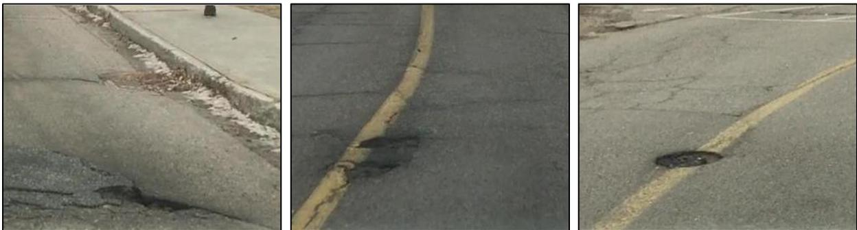
**Figure 5. Examples of potholes on paved roads**
