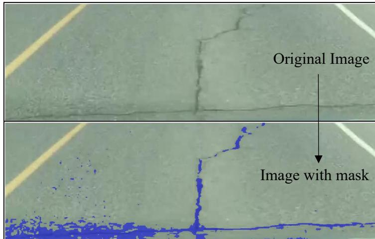
**Figure 31. An image of a crack in the road and a threshold mask laid on top of it**
