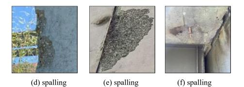
Figure 4.3: Sample images for defects dataset (a, b, c) crack and (d, e, f) spalling (Image Courtesy: TBT Engineering)
