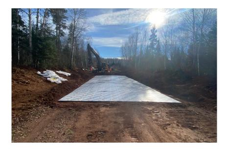
Figure 3. Southbound view of test section 1 prior to covering the insulating layer.
