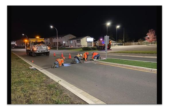
Figure A14: Installing the strips on the pavement.
