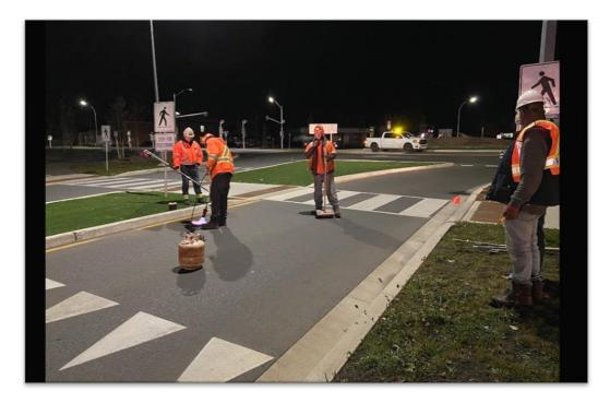
Figure A13: Cleaning the surface with a broom, followed by drying the surface with a blow torch before installing the strips at about 5 am local time on Thursday, October 27, 2022
