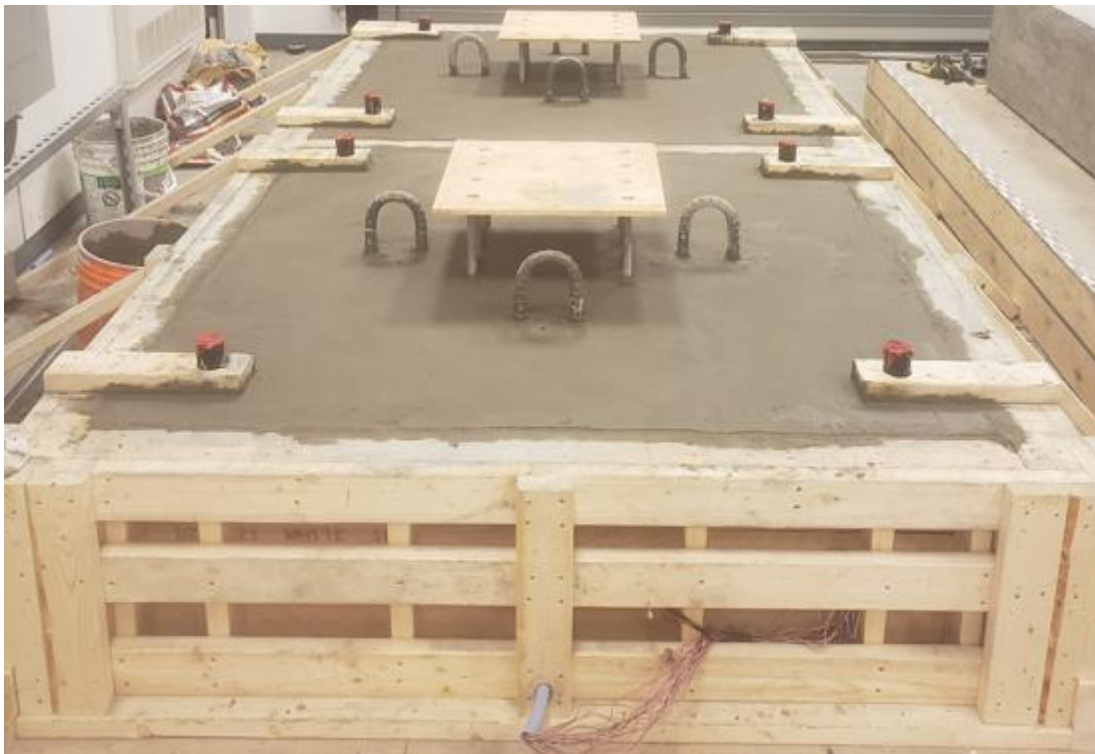
Figure 8 Concrete Pedestal Forms After Pour
