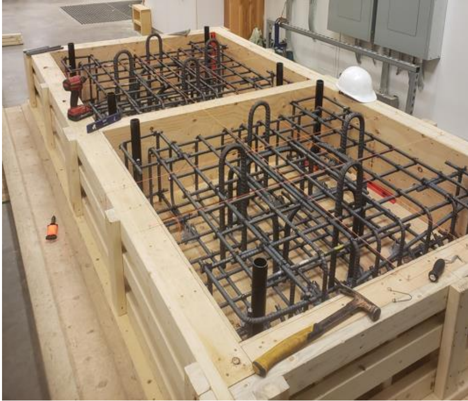
Figure 7 Concrete Pedestal Forms Before Pour
