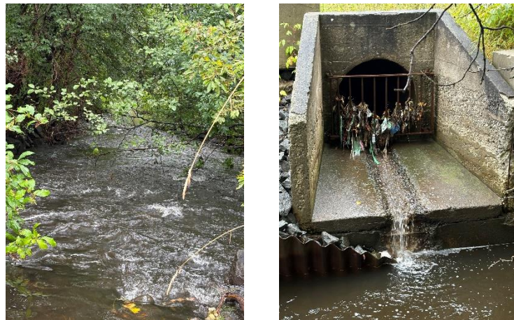
Figure 5-6 Stream reach and stormwater outfall at Site 4.
