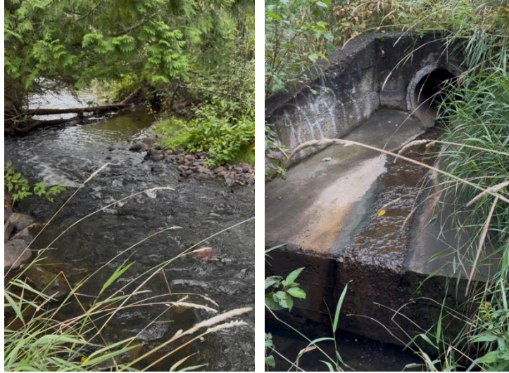
Figure 5-4 Stream reach and outfall at Site 2.
