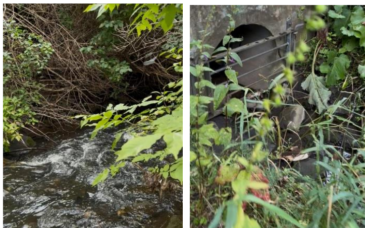
Figure 5-5 Stream reach and outfall at Site 3.
