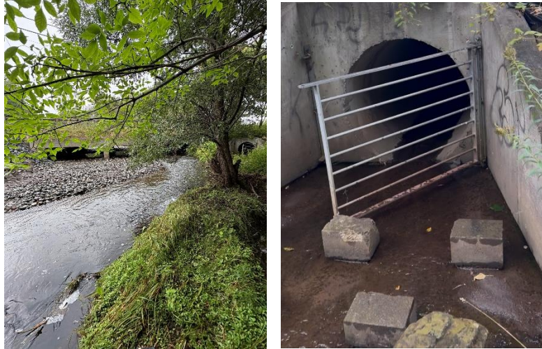
Figure 5-7 Stream reach and outfall at Site 5.
