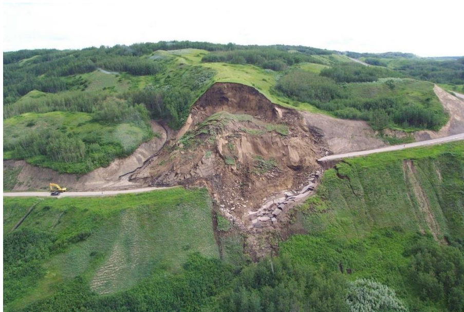
Figure 1.1. Cecil Lake road landslide, Peace River (Couture et al. 2013)
