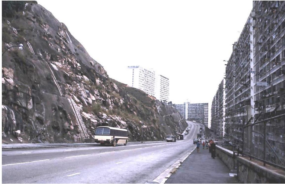
Figure 4.3. A view down Sau Mau Ping Road in Kowloon showing apartment blocks across the road from the steep rock slopes (Hoek and Bray, 1974)
