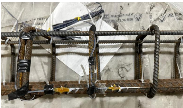
Figure 6.13: Strain gauge installation
