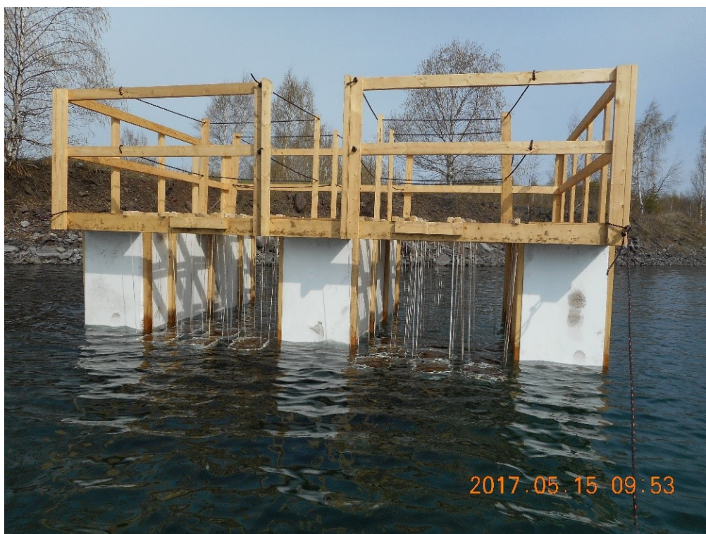
Figure 3.6. Configuration of raft assemblies deployed in pairs in the three legacy-mine influenced pits. No wire-mesh encasements for individual quadrats were used on these rafts.
