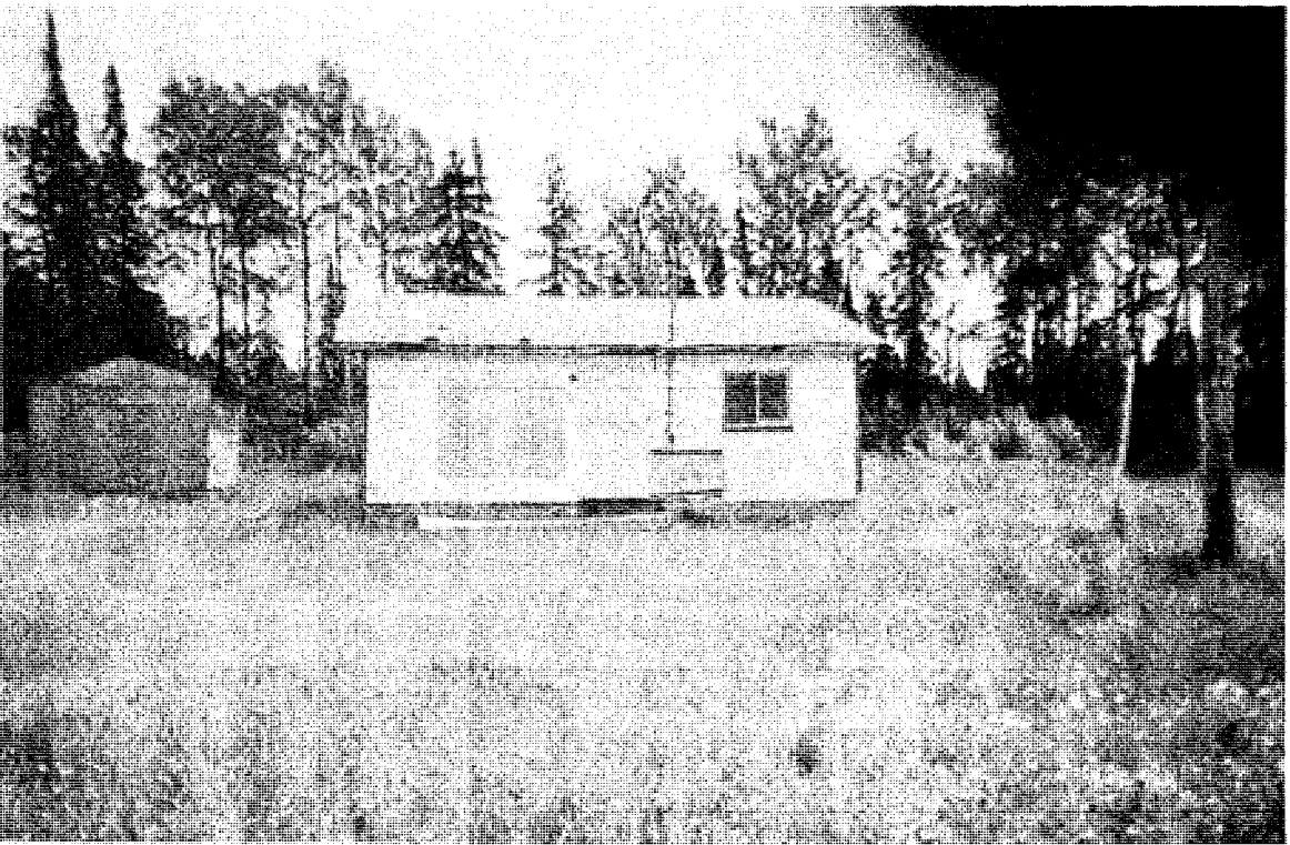
Figure 11. Picture of a condemned house in the community.
