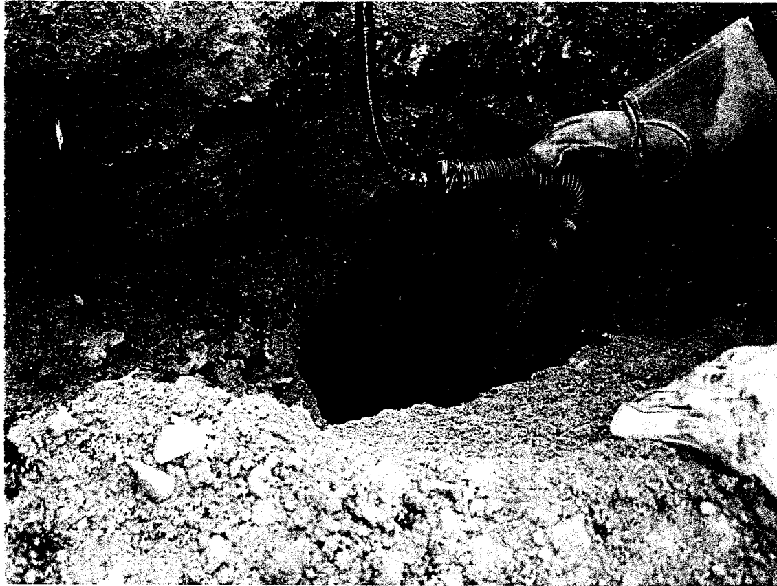
Figure 3.3 Thermistor Installation at Northeastern Study Site
