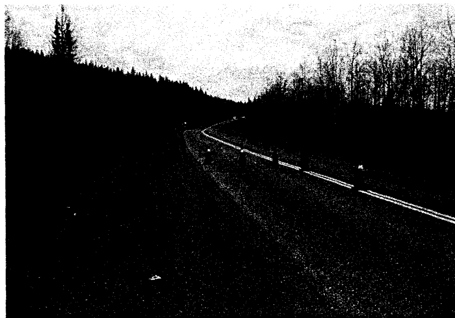
Figure 3.13 Highway 527 Study Site
