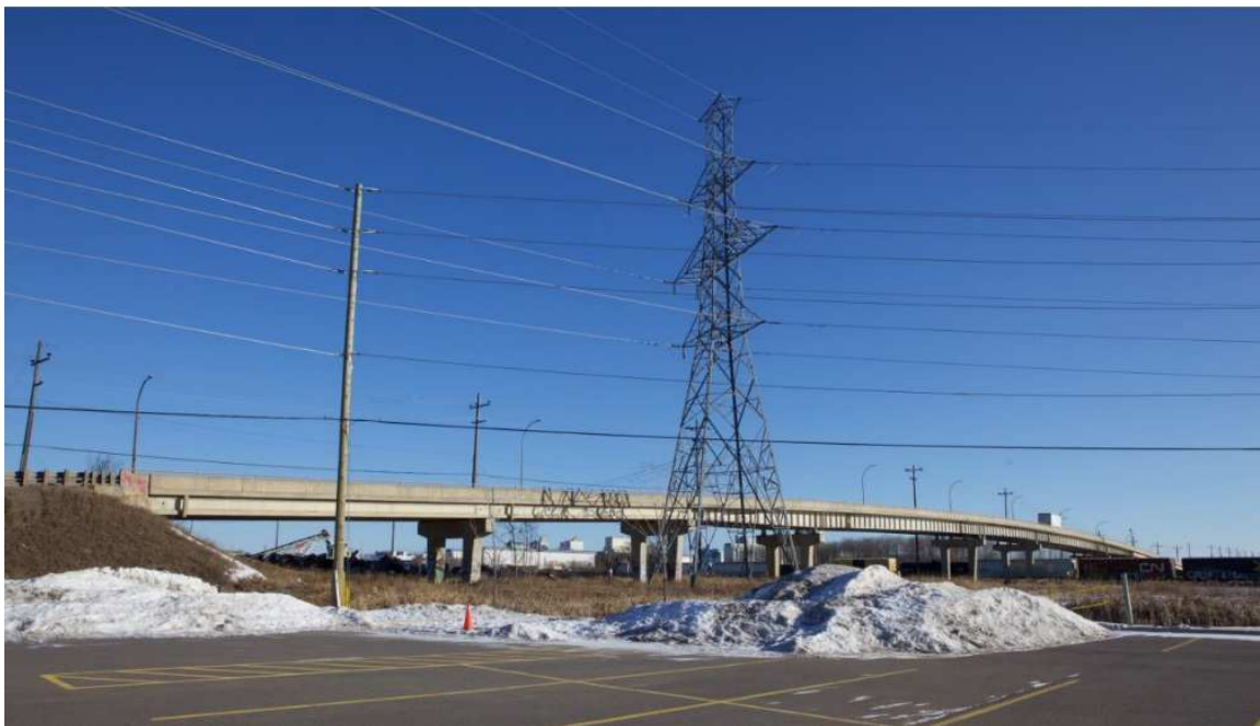
Figure 4.11: Long-span bridge in Thunder Bay
