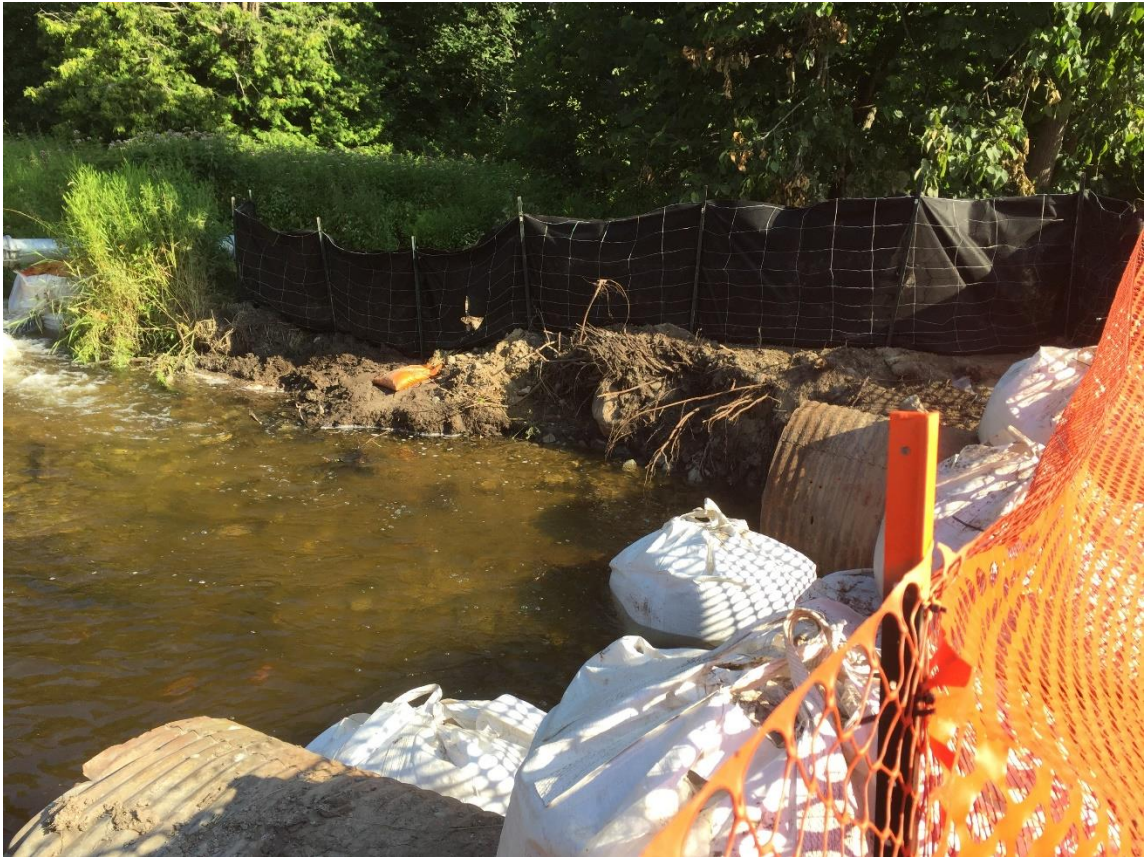
Figure 3. View of metal culverts as prepping for extraction begins (Ewaskiw 2017)
