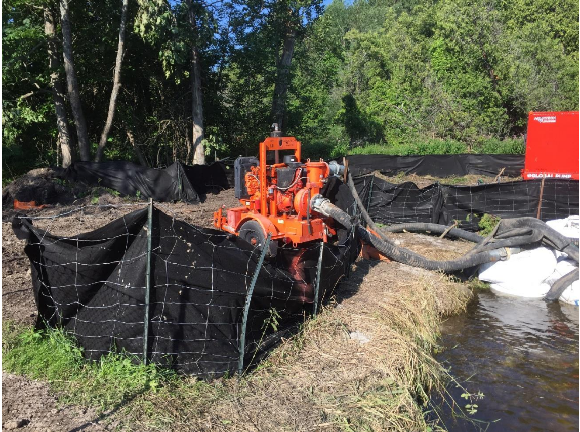
Figure 2. Water pump from culvert extraction site at Albion Hills (Ewaskiw 2017)
