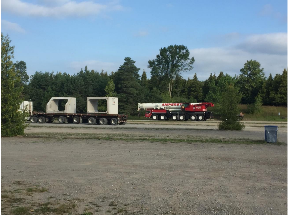
Figure 6. View of concrete culvers prior to installation (Ewaskiw 2017)
