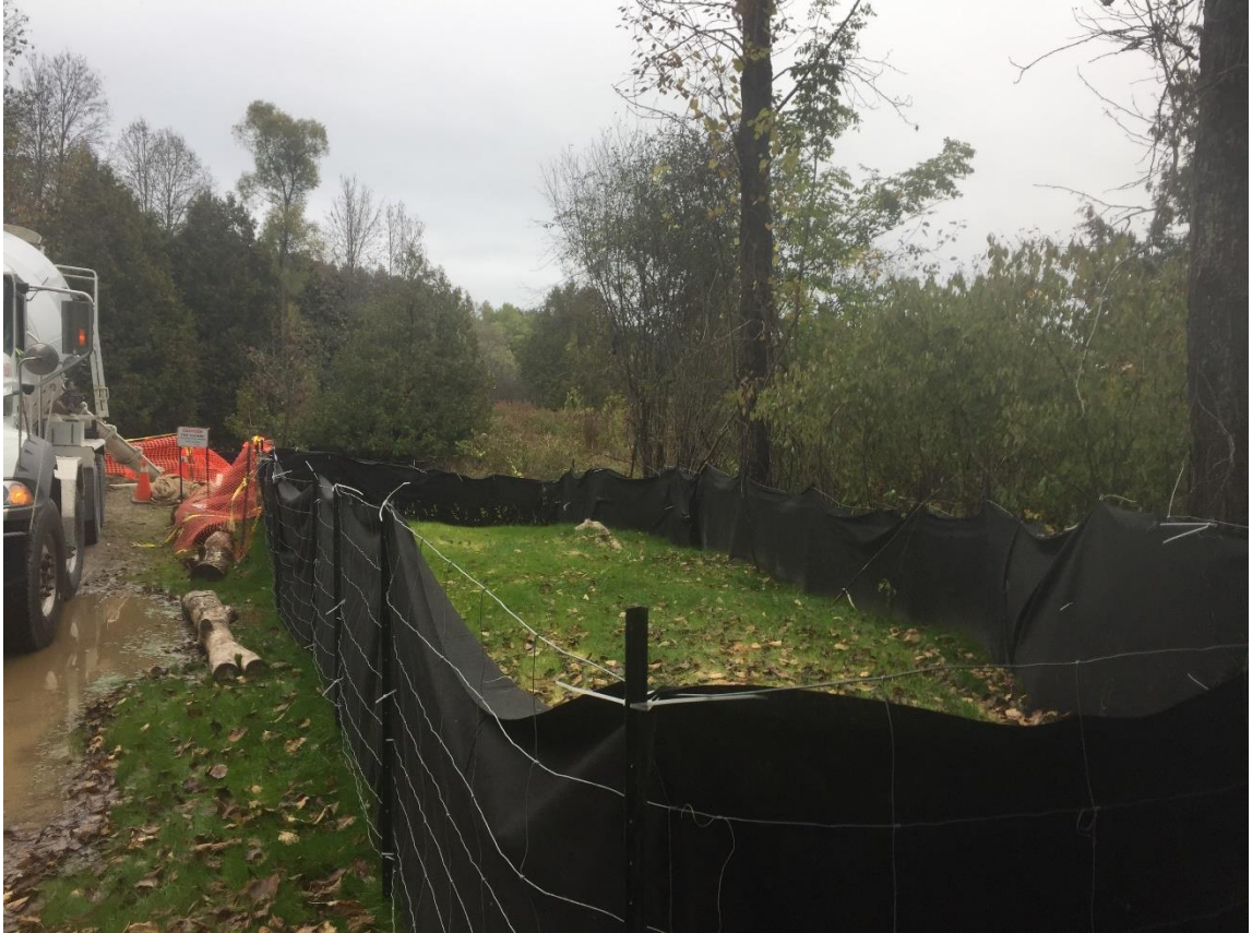
Figure 7. Riparian preservation with silt fences (Ewaskie 2018)
