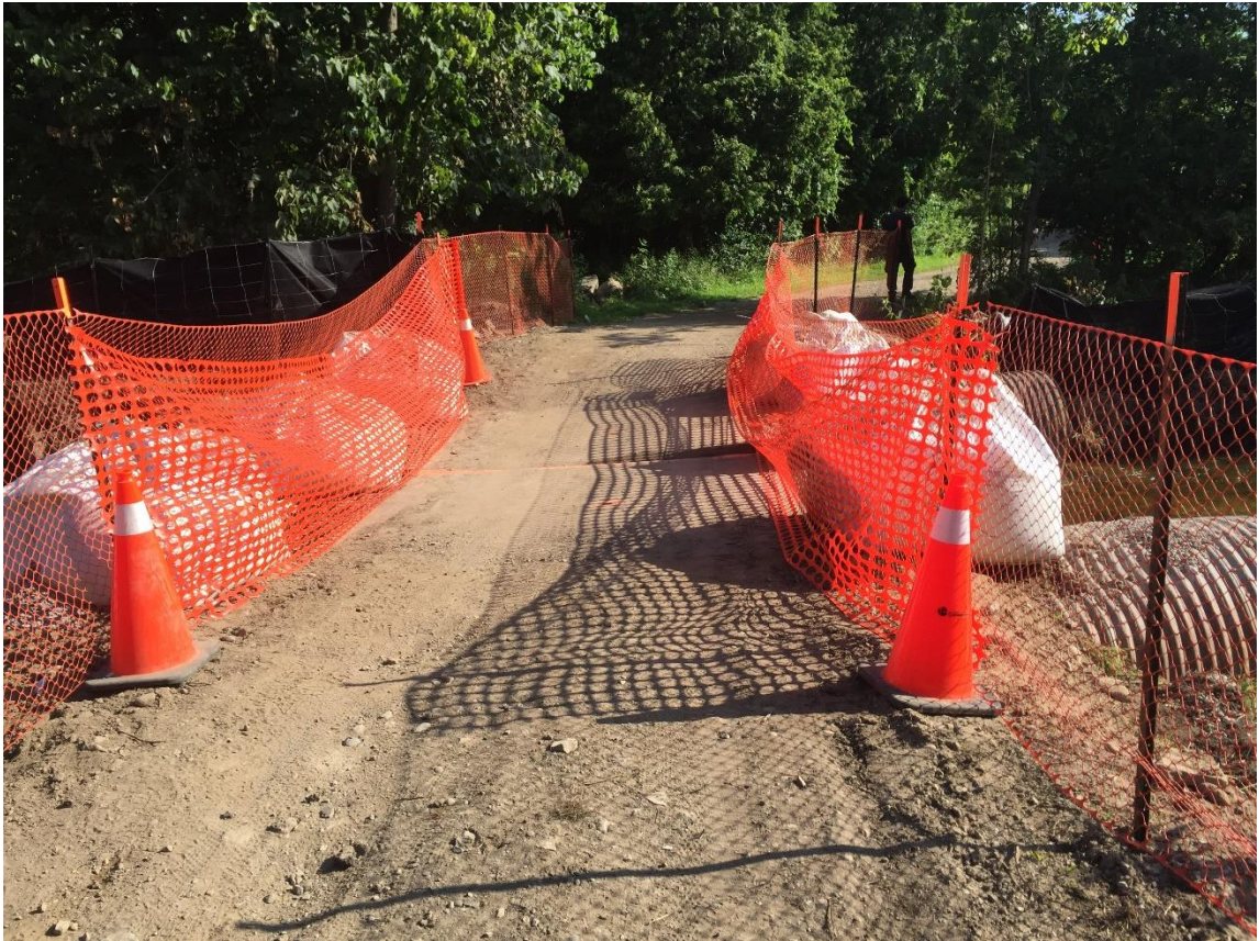
Figure 4. View of roadway water crossing prior to culvert extraction (Ewaskiw 2017)
