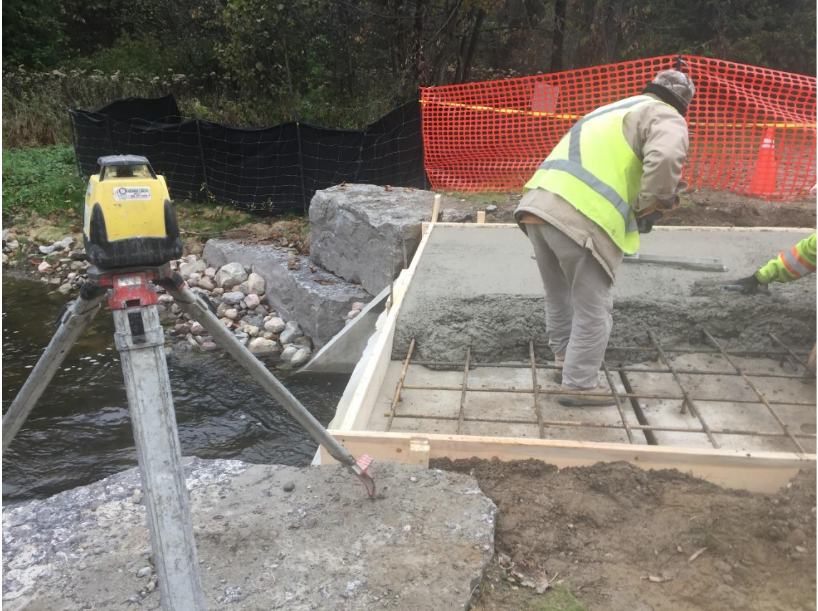
Figure 8. View of setting the concrete culvert (Ewaskiw 2018)
