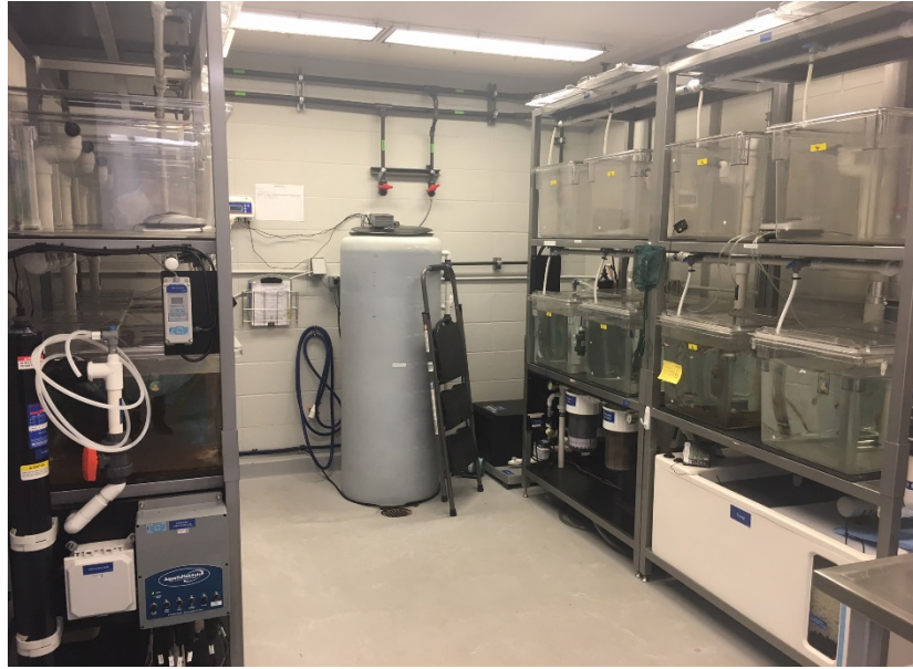
Figure 4. Tanks inside the Aquatic facility housing numerous fish species. Filtration systems can be seen towards the bottom left and bottom right (Rugo 2018).
