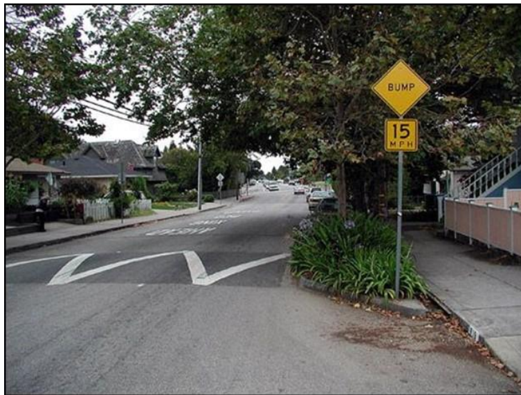
Figure 6.23: A speed hump placed along a local residential road (NACTO, 2013).
