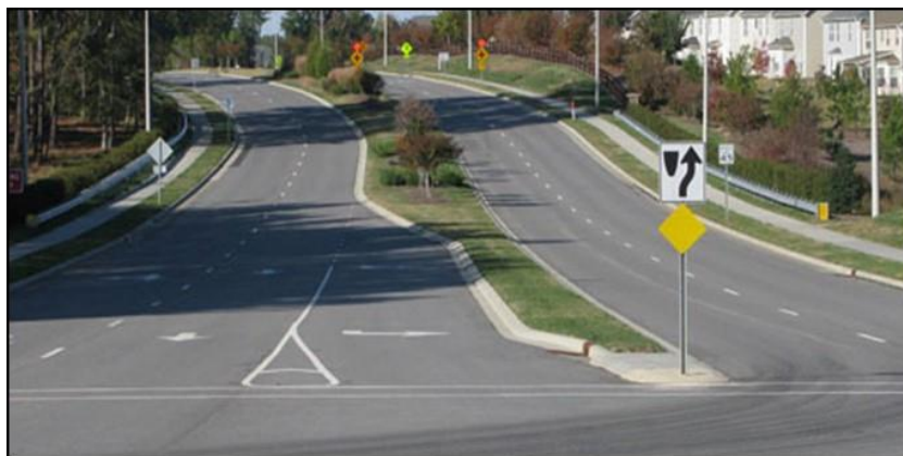
Figure 6.26: Roadway with a physical median (FHWA, 2016).
