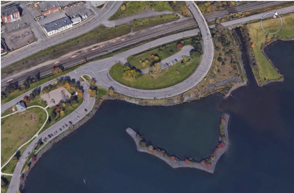
Figure 45: Sanctuary Island and Howe Street Overpass.
