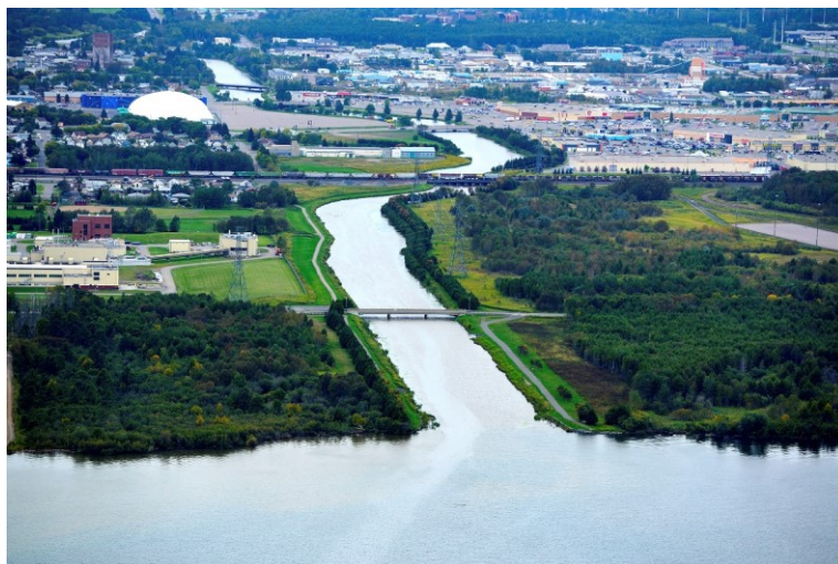
Figure 8: Aerial View of the Neebing-McIntyre Floodway (Lakehead Regional Conservational Authority, 2019).
