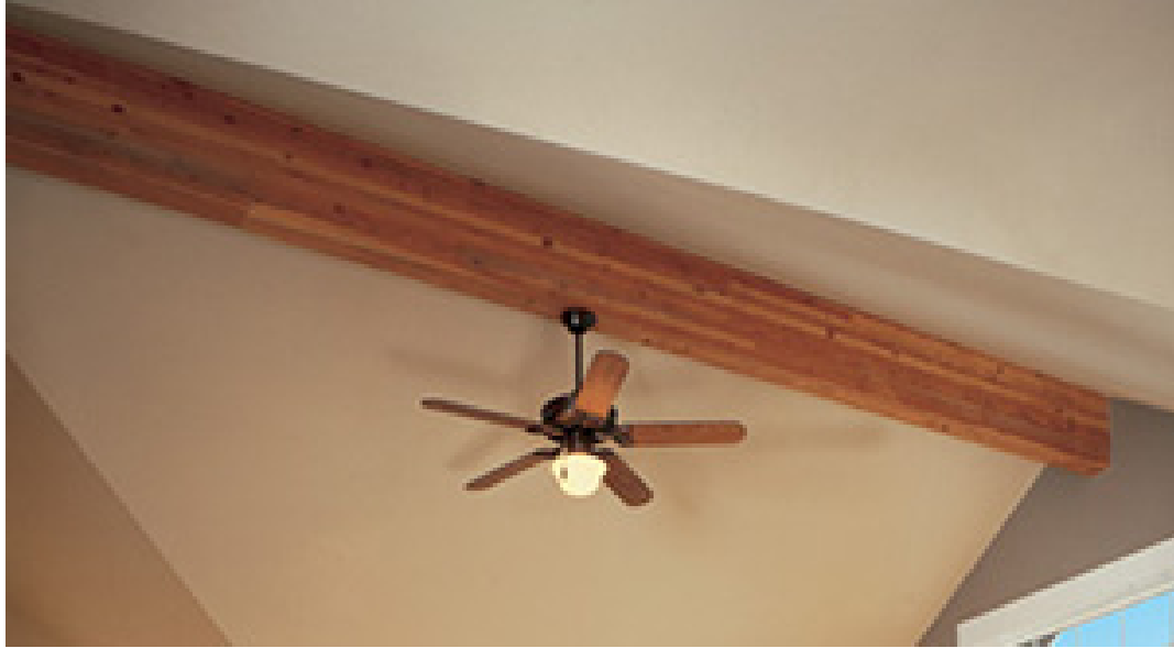
Figure 16. A Glulam beam utilized as a Ridge beam to create a high ceiling and raise the aesthetics of a room (APA 2021).
