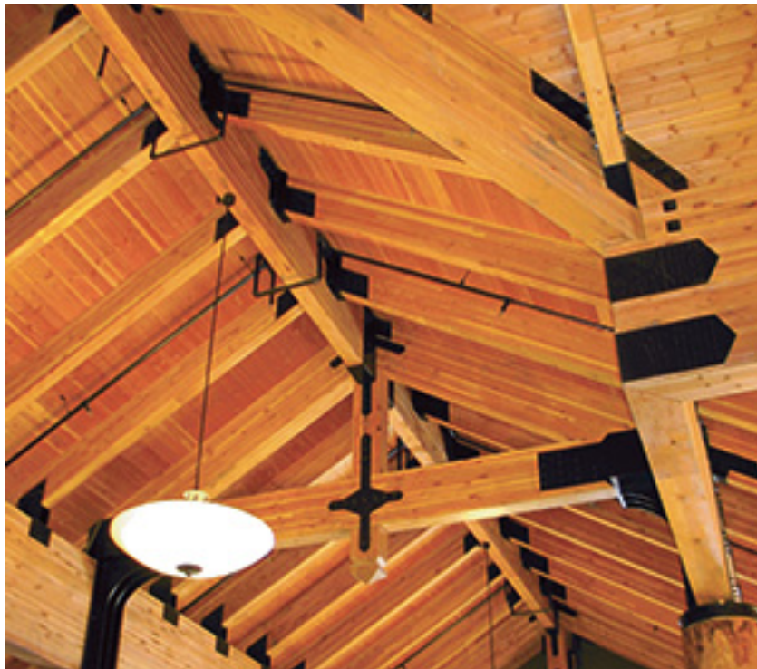
Figure 15. Vaulted ceilings created from Glulam beams and rafters (APA 2021).
