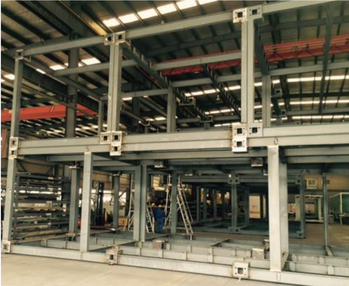
Figure 2.21 Steel connection assembled (Hwan Doh et al., 2017)
