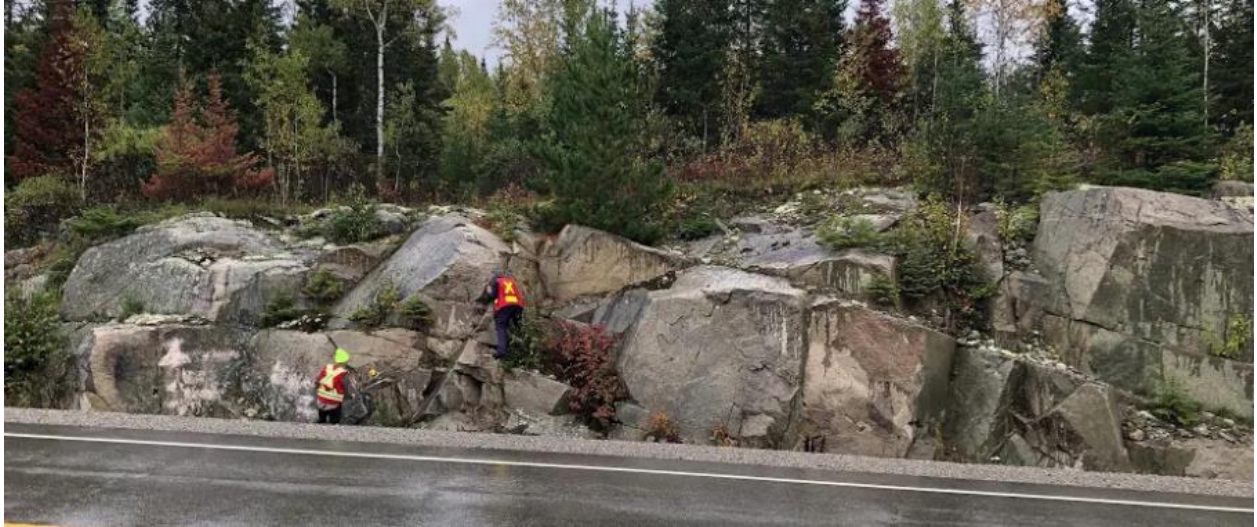
Figure 12. The Sabaskong batholith outcrop located along Highway 71. The steeply dipping fractures are chlorite and/or epidote infilled shear fractures while most of the sub-horizontal fractures are unfilled.
