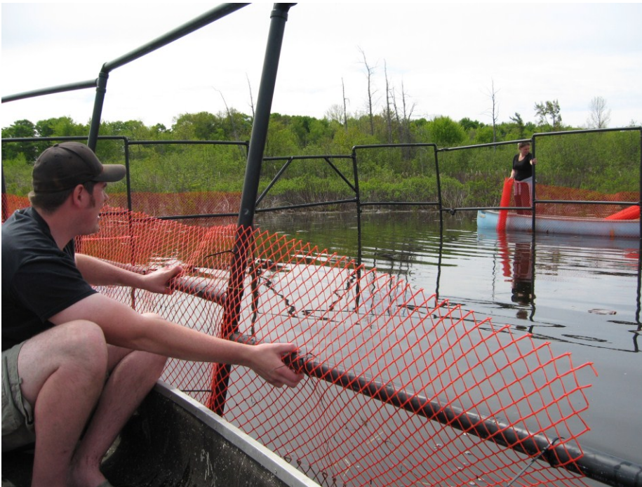
Figure B.4.2 – Victoria Point fence installation.
