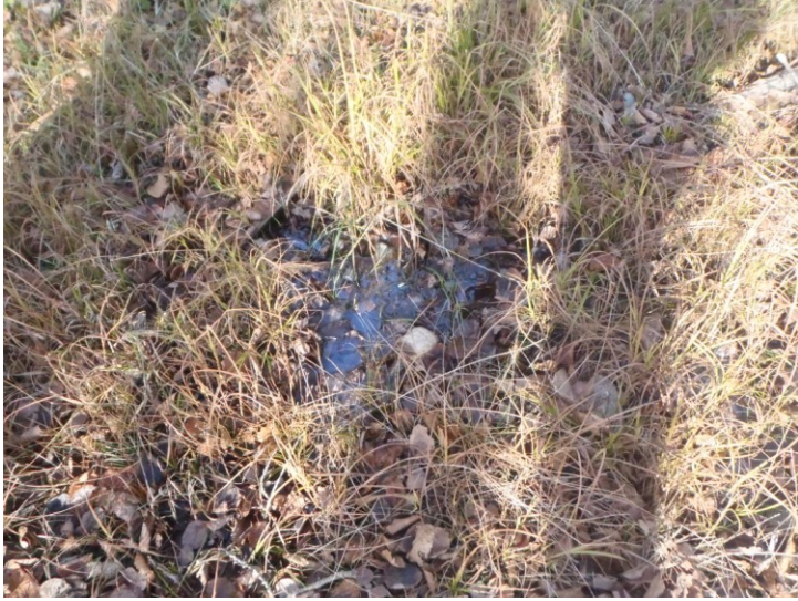
Figure 4.2a Groundwater seep located on the bank of newly restored reach of Kama Creek.
