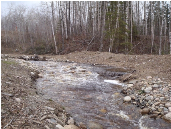
Figure 4.14c. 2014 new channel showing erosion of banks.
