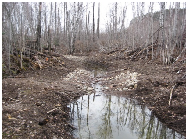
Figure 4.9b. Little deposition in 2012 as channel was freshly dug
