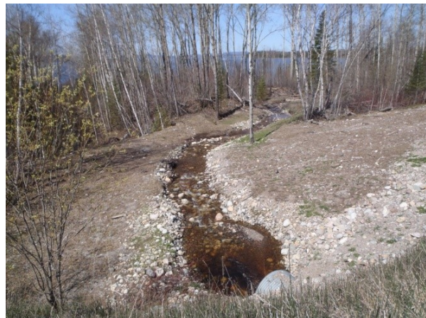
Figure 4.13b. New channel in 2014, constructed in pre 1960's 'natural' channel.
