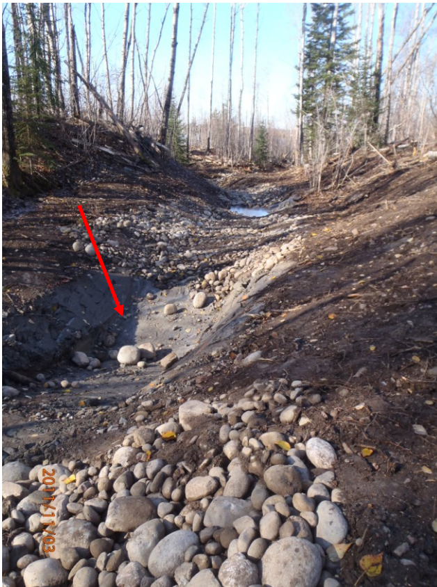
Figure 4.2b and c. Photos of clay bottom found when excavating reach 2 of Kama Creek. Arrow points to thick clay layer in pool of new channel (left). On the right, section of clay showing layering.
