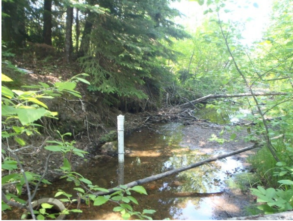
Figure 4.14a. 2011 old channel showing steep eroded banks.
