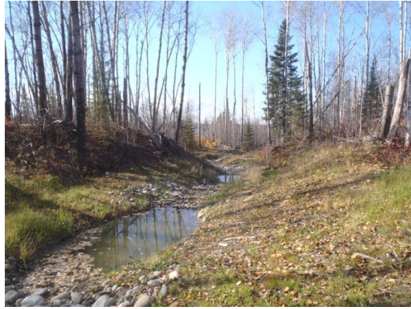
Figure 4.14b. 2012 new channel showing little erosion on banks.
