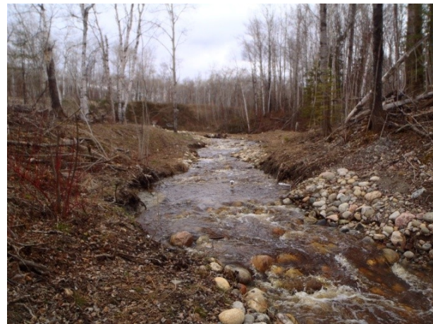
Figure 4.12b. Optimal occurrence of riffles in new channel.
