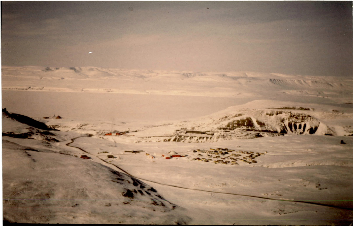
NANISIVIK MINE SITE. FROM FRONT TO BACK; TOWN SITE , WEST OPEN PIT WITH ADIT (RIGHT) AND MILL (LEFT) , DOCK FACILITY (FAR LEFT) , AND STRATHCONA SOUND
