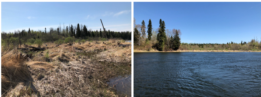
Figure 4.1: Nipigon River landslide area (2018)
