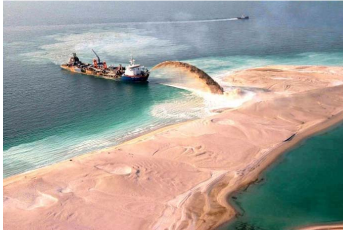
Figure 1.1 Palm Islands construction in Dubai
