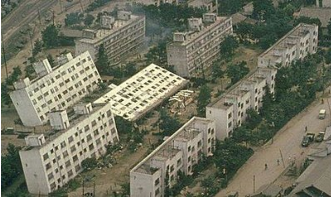
Figure 1.1: Soil liquefaction at Niigata (Vukobratovic and Ladjinovic, 2013)
