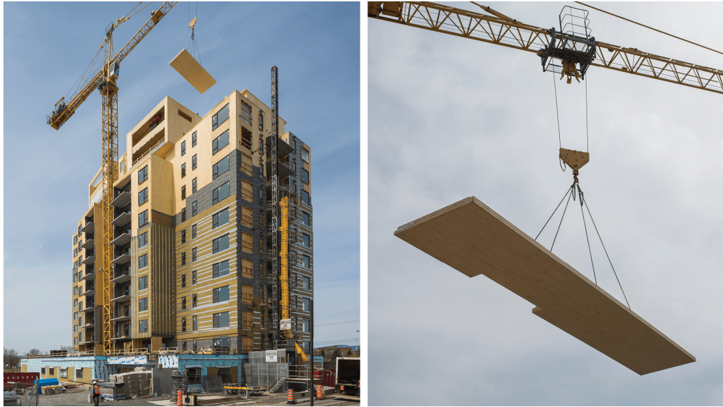
Figure 5: Project of Origine under construction. (Source from: Nordic Structures http://nordic.ca/ )
