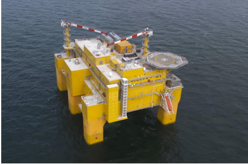
Fig. 1-3 “Dolwin2” offshore substation [3].
