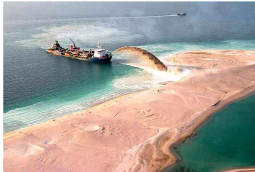
Figure 1.3: Palm Islands construction by oblique discharge of slurry jet.
