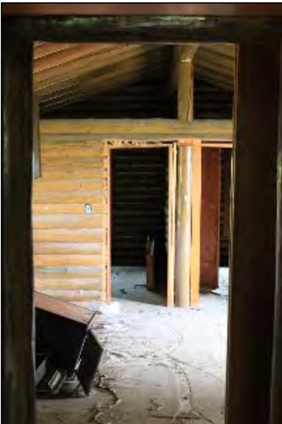
Figure 6.36, School Teachers Residence as viewed from interior. Grouting used as chinking, multiple preplanned rooms with doors, electric wiring not exposed, finished and varnished logs.
