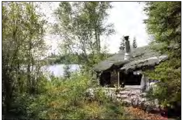
Figure 6.41, Cabin 3 facing south.
