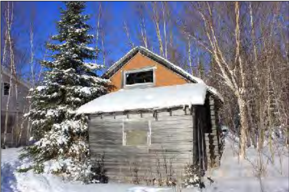
Plate E.11, Old schoolhouse facing north.
