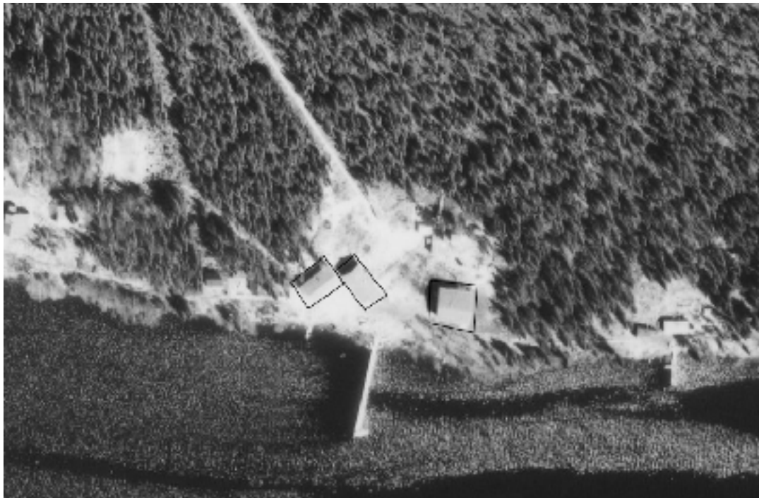
Figure 6.33, Aerial imagery of the Provincial school and the teachers and principals accommodations (National Air Photo Library 1986).
