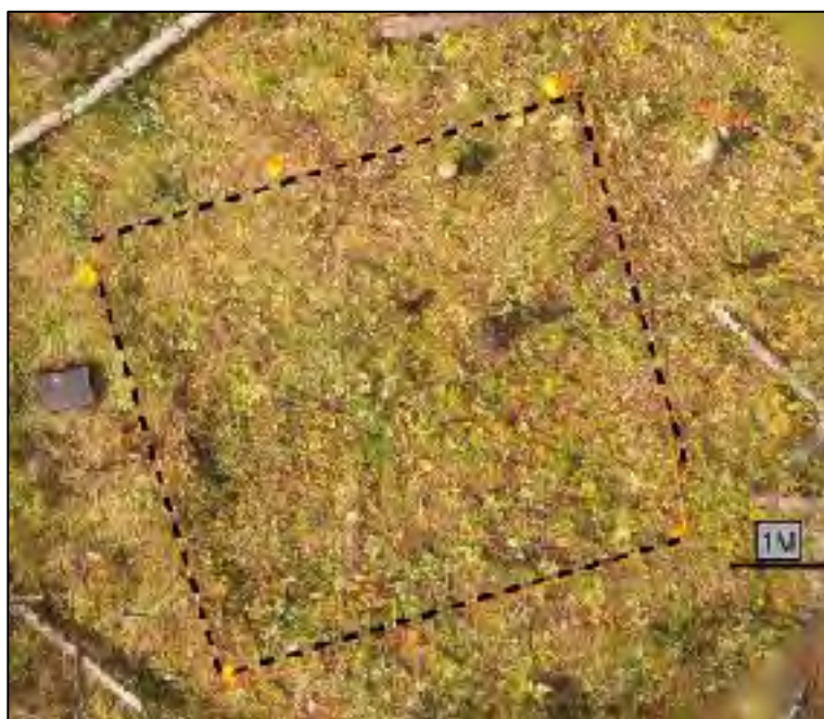
Figure 6.6, Sams Cabin overview as taken by drone, the outline of the cabin foundation is traced in black.
