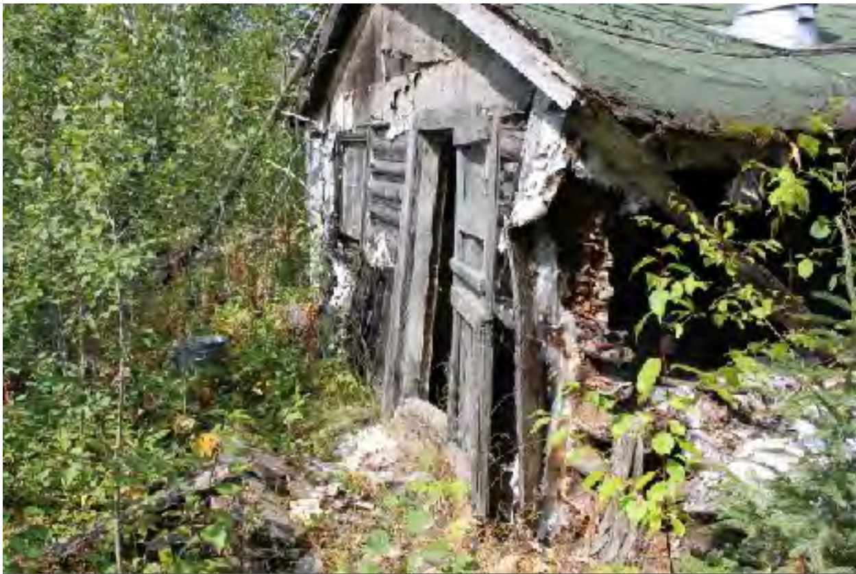
Figure 6.43, Photograph of Cabin 3 facing northwest.
