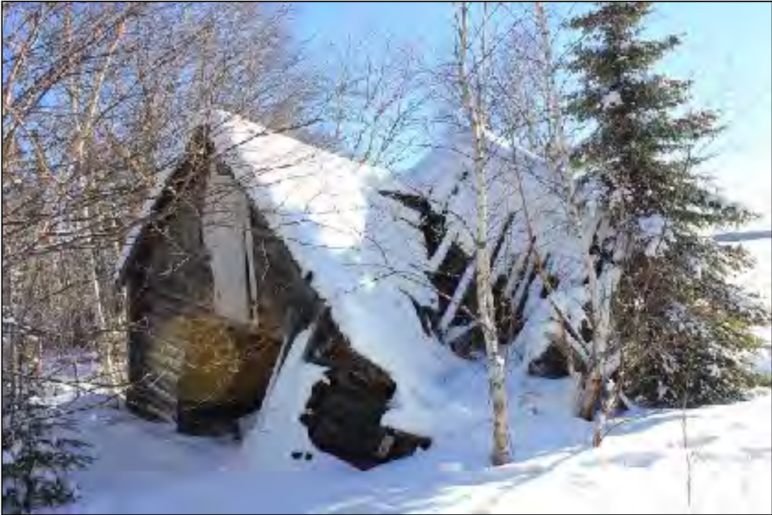
Plate E.10, Old schoolhouse facing south.
