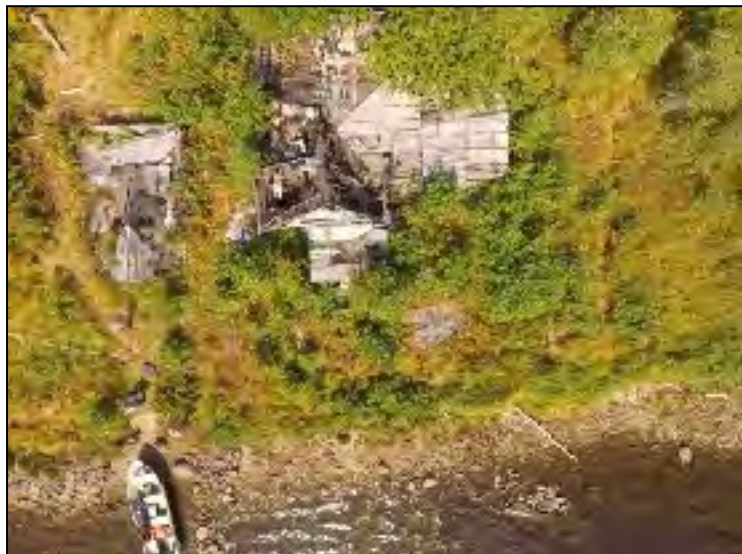
Plate E.29, Over flight photo of Cabin 8 by drone.
