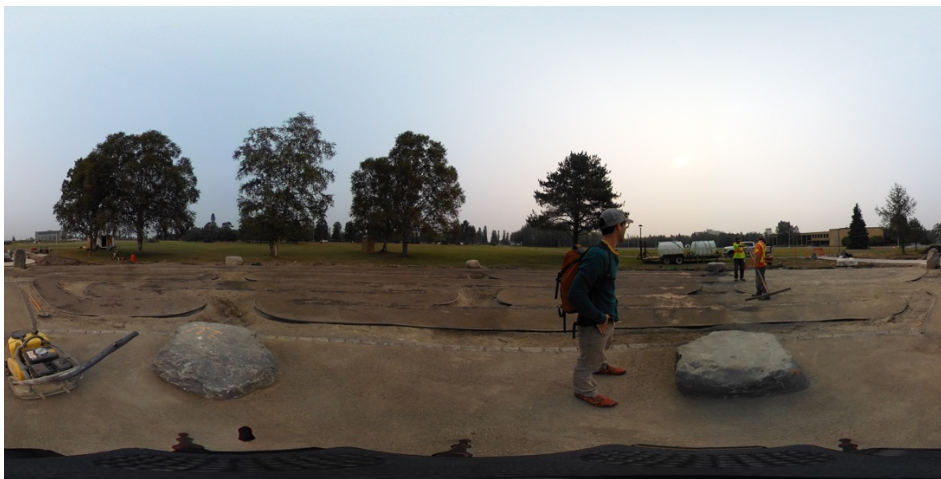
Figure 11. 360-degree image of Lakehead Wellness Path Labyrinth Construction Aug 4 th , 2021
