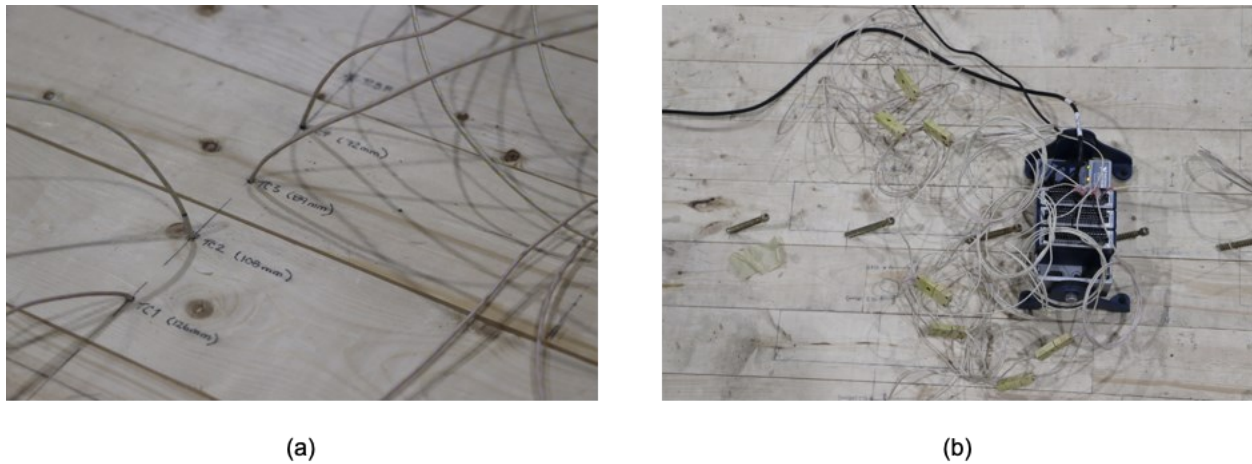
Figure 3.13: Thermocouple installation process.
