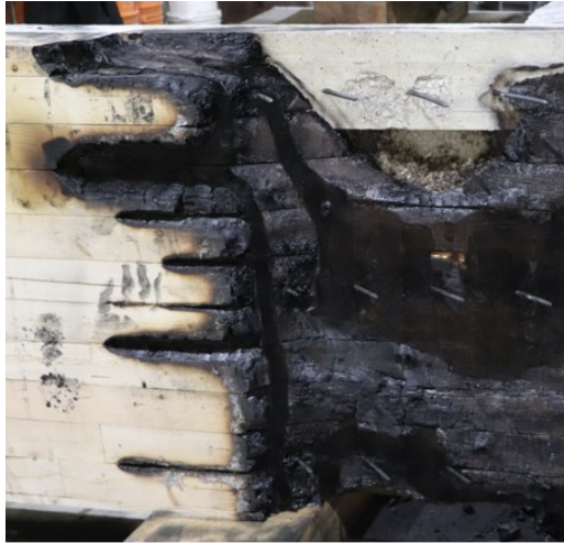
(a) Slab 1 - Left Side
