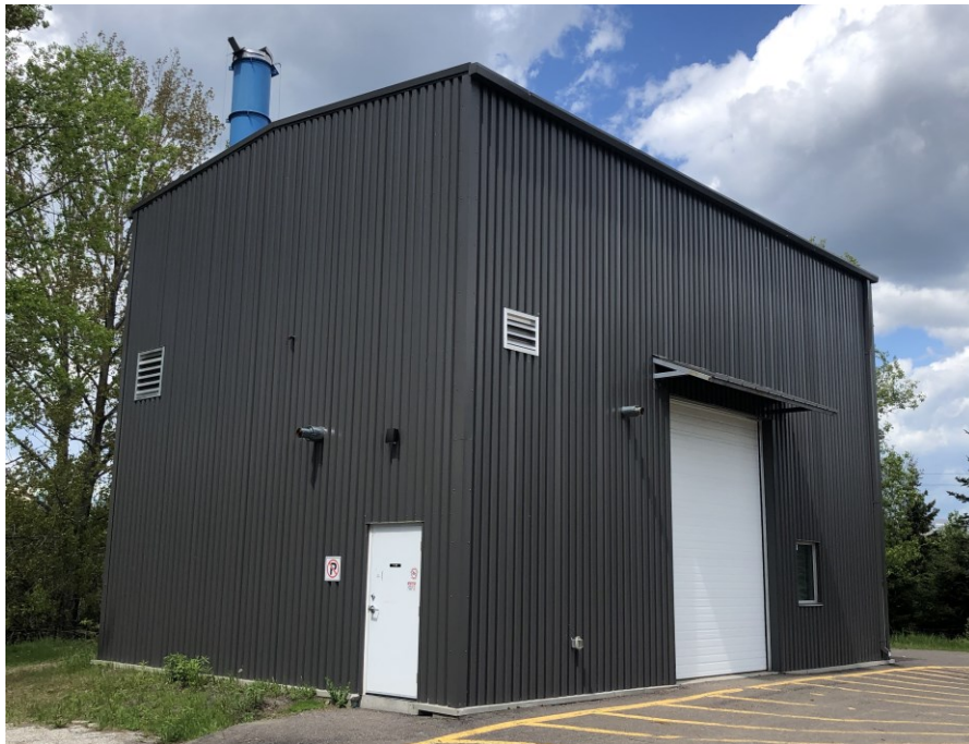
Figure 3.1: Lakehead University Fire Testing and Research Laboratory – LUFTRL (Courtesy of Dr. Salem).
